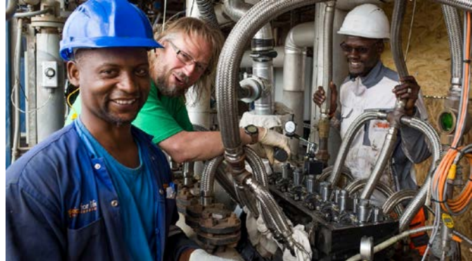
Technicians Working on New Engine
