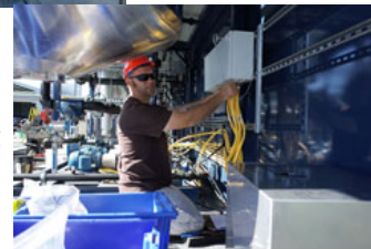
Connecting cables to the pump sled control panel
