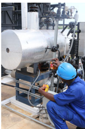
Senegalese worker performing maintenance tasks on the JOP
