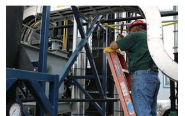
Fitting and installing pipe spools
