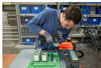
Constructing one of the boiler control panels
