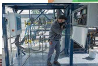
Mounting the steam distribution control panel
